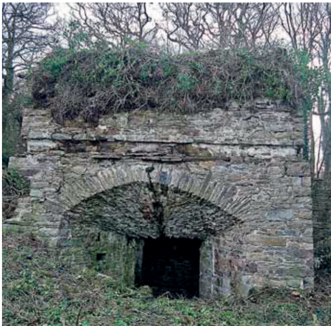
Eighteenth-century blast furnace at Bealkelly, Co. Clare
